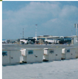
4 Apojet units, Malpensa Airport, Italy
