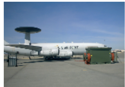
Piller equipment at AWACS bases worldwide
